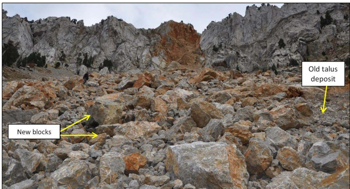
Fig. 4: View of the lower zone of the YDC. Almost continuous debris cover generated by the Vilanova de Banat rockfall, lying on a previously existing talus deposit. New blocks stand out from the old ones by their most vivid colours (reddish, yellowish). Distinct fresh fractures and spalling as a consequence of the impacts are also observed.
