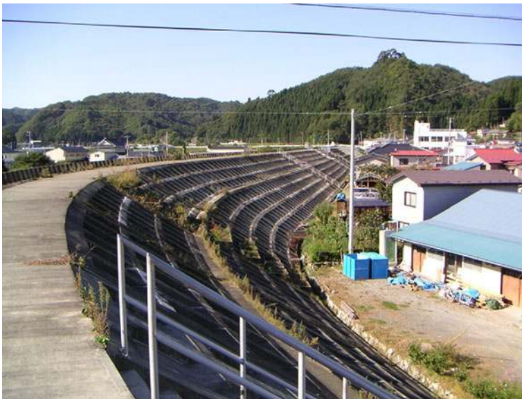
Fig. 8 Ten meter high coastal dykes in Taro, Miyako City (Before the tsunami; Ministry of Land, Infrastructure, Transport and Tourism)
