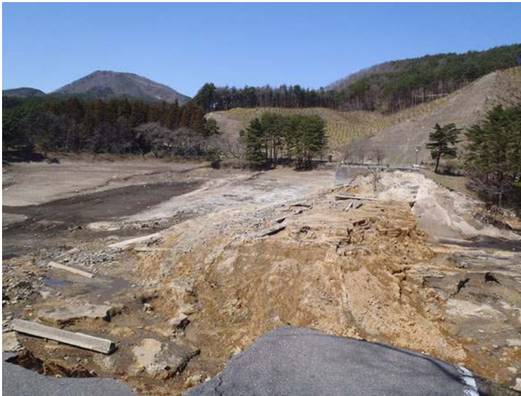
Fig. 4 Burst dam (Fujinuma reservoir)
