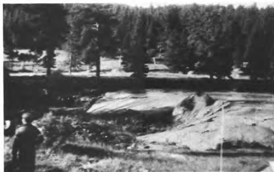
Figure 6. Photographs showing sequence of Cascade Lake Dam failure, Colorado, July 15, 1982 (from Jarrett and Costa, 1985).
