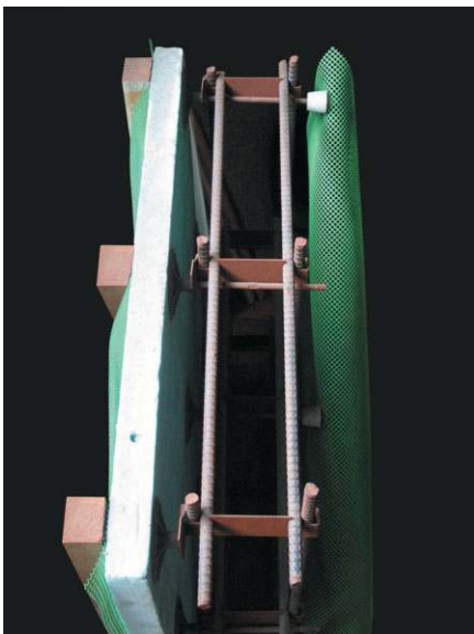
Fig. 13. Zero-waste formwork by Kenzo Unno and resulting wall in the “URC house with grass” in Edogawa-Ku, Tokyo, Japan (2003)
