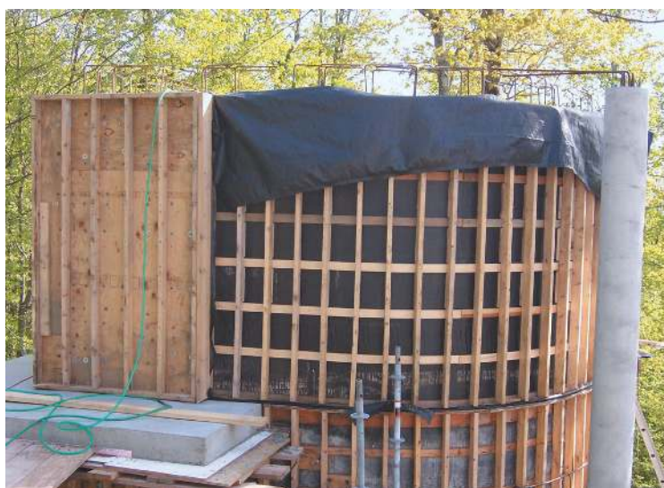
Fig. 15. Black Tree House (2007) during construction of fabric-formed walls and columns, and after completion. Reproduced by permission of Arro Design, Sandy Lawton
