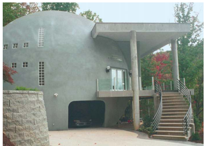
Fig. 18. Cloud Hidden house, built using pneumatic formwork (2000). Reproduced by permission of the Monolithic Dome Institute
