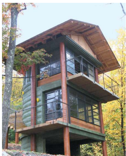
Fig. 15. Black Tree House (2007) during construction of fabric-formed walls and columns, and after completion. Reproduced by permission of Arro Design, Sandy Lawton
