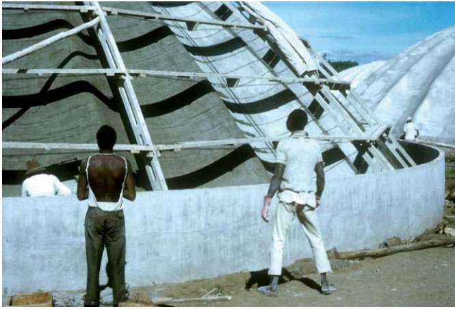
Fig. 9. A Cyprus bin under construction in Nakuru, Kenya (photo by Grant Maslen). Reproduced by permission of Hilary Hann
