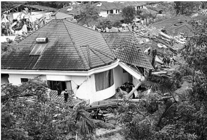
Figure 2. 2008 Bukit Antarabangsa Landslide [25]
