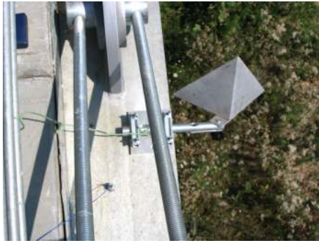
FIGURE 4: Corner reflector installed on a bridge.
