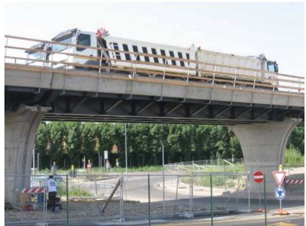
FIGURE 12: Testing of a bridge.
