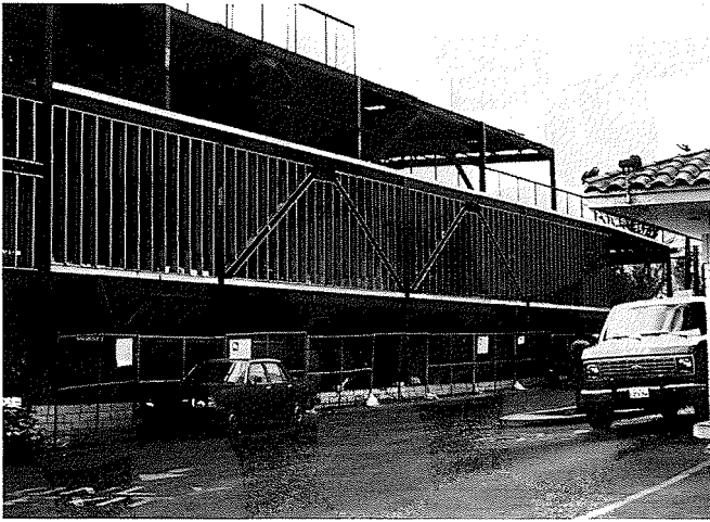
Fig. 12. Three-storey building under construction in Van Nuys: chevron bracing on the north wall.
