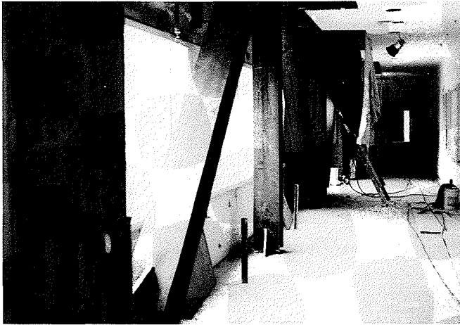
Fig. 30. Four-storey commercial office structure: newly installed braces in repaired inverted chevron-type braced-frame with vertical tie-members added to implement “zipper” system.
