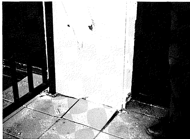
Fig. 6. First Interstate Bank Building in Northridge: column uplift at the base of the X-bracing.
