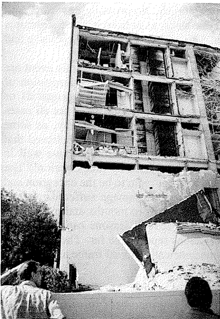
Fig. 38. Van Nuys office building: end wall failure on east face of building.
