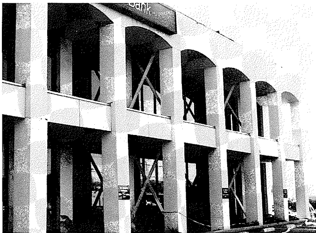
Fig. 4. First Interstate Bank Building in Northridge: steel X-bracing in the facade.
