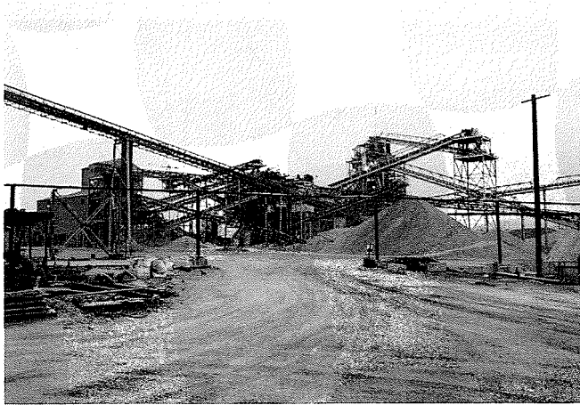
Fig. 19. Asphalt and rock plant: typical conveyor and truss system.
