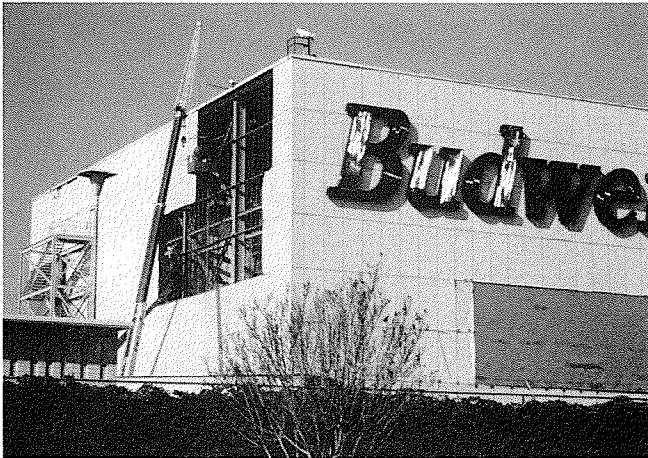
Fig. 16. No. 2 Brewhouse, Anheuser-Busch, Inc.: global view of cladding failure on warehouse.
