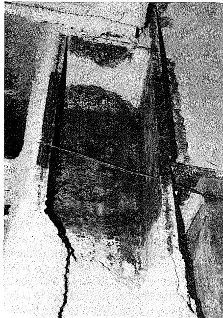
Fig. 40. Moment resisting frame under construction: typical beam-column connection damaged by column cracking and fracture at the level of the beam's lower flange weld.
