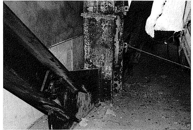
Fig. 29. Four-storey commercial office structure: close-up view of new gussets at brace end for corner columns.
