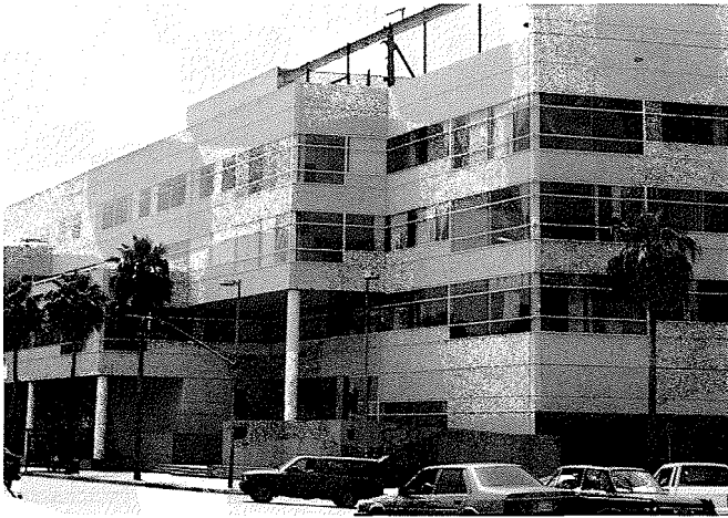
Fig. 22. Four-storey commercial office structure: global view.
