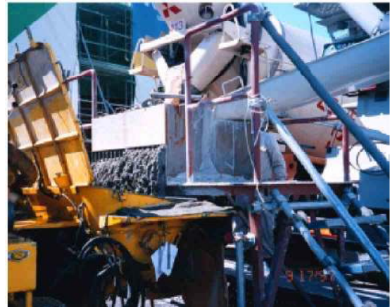
Fig. 25 Automatic acceptance test at job site.
