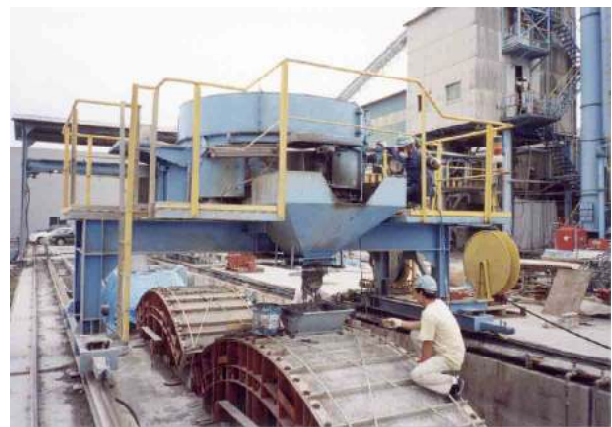
Fig. 32 Casting of SCC for Tunnel Segment.
