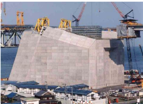
Fig. 31 Anchorage 4A of Akashi-Kaikyo bridge.
