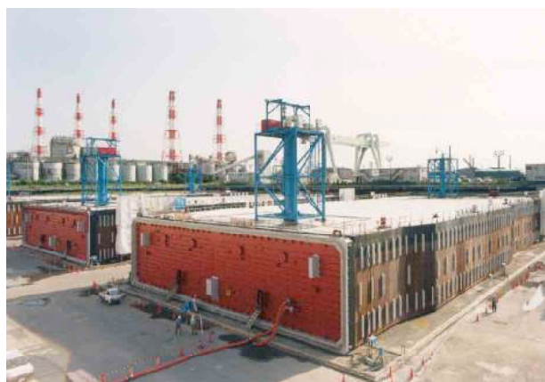
Fig. 35 Sandwich structure for immersed tunnel.
