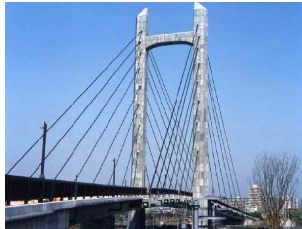
Fig. 29 Shin-kiba Ohashi bridge.
